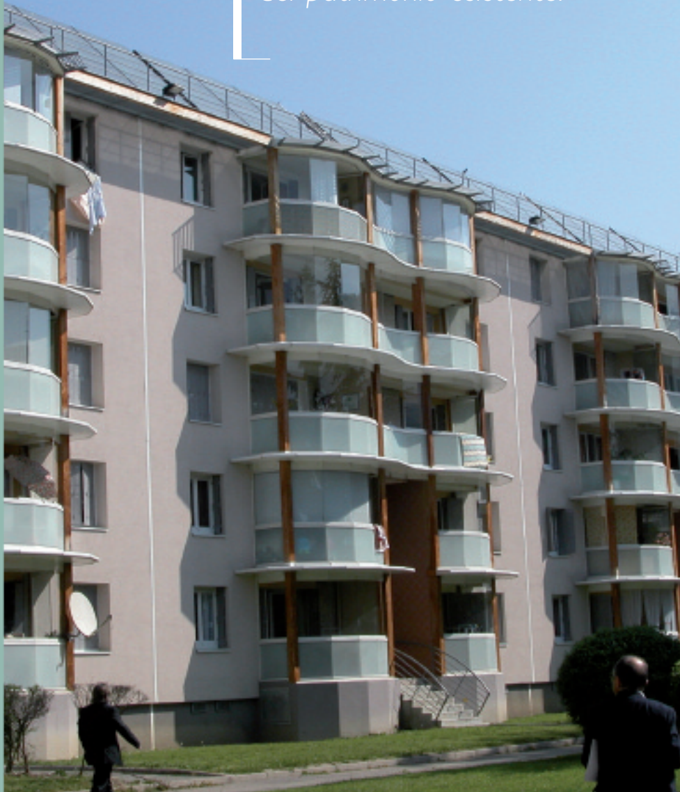
Fig. 5 - France-St. Martin d'Heres- 2006 Retrofitting of 360 social dwellings promoters: OPAC38 co-financed by the EC- SUNRISE project
